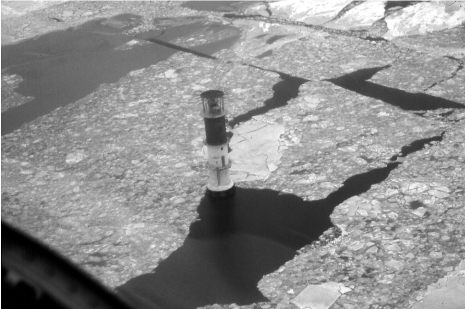
Figure 5.1 Sea ice drifts pass the lighthouse Nahkiainen, northern Baltic Sea. The width of the lighthouse is about 5 m.
