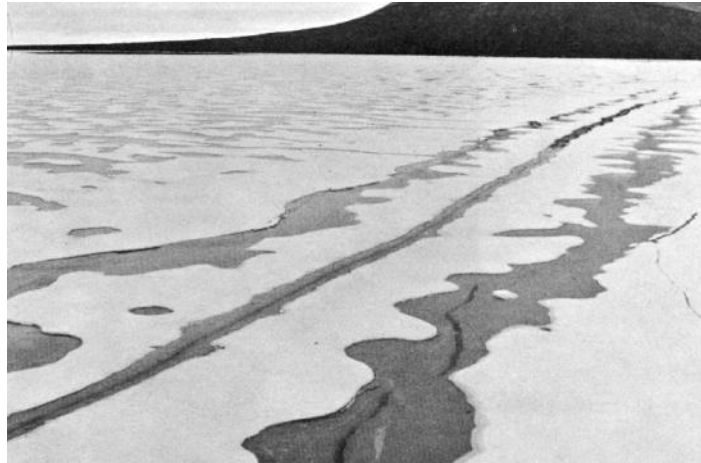
7.1.1 Crack (Fissure [fr]) Defence Research Boat, Canada
